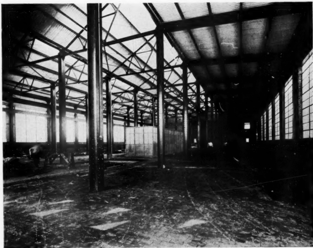
PLATE 16 BUILDING FOR BALTIMORE OIL ENGINE CO., BALTIMORE, MD. WALTER M. GIESKE, ARCHITECT
