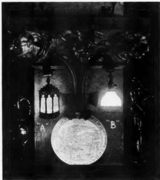
Fig. 4.—For economic reasons it was considered necessary to install shades like "B," which are as common as dirt and equally attractive. An ideal design to harmonize with the fixture and its ground is illustrated ("A"), but the expense of reproducing this lantern in quantity was slightly in excess of the appropriation. Fig. 5 shows the result of searching the commercial market in the attempt to approximate the desired ideal, usually a hopeless task, but in this particular instance the "exception" ruled.
