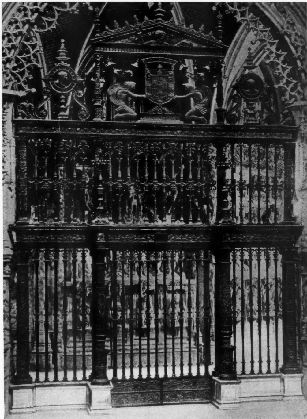
WROUGHT IRON REJA, CONSTABLE'S CHAPEL, BURGOS CATHEDRAL (From Rejería of the Spanish Renaissance)
