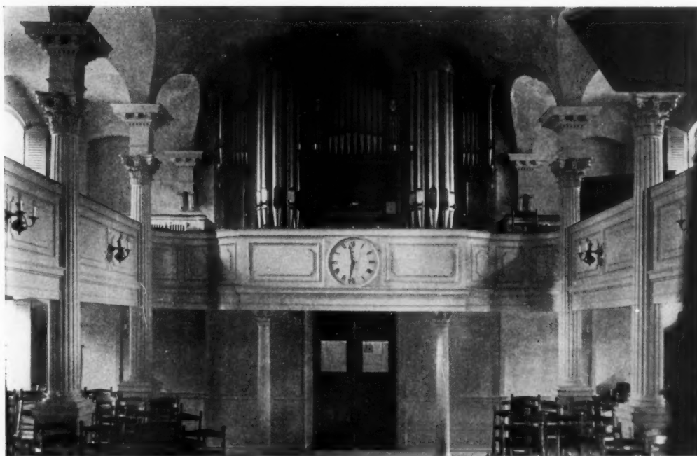
INTERIOR OF ALL SOULS CHURCH IN THE EAST, SUMMIT, N. J. Looking from chancel. The Renaissance organ, with colonial recessed console, recently installed
