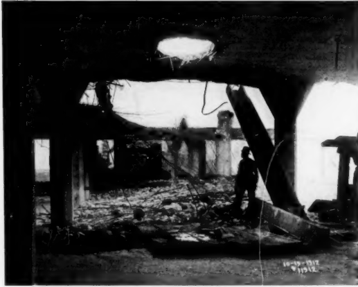
THE HOLE IN THE CEILING SHOWS THE ONLY EFFECT PRODUCED BY THE DROPPING OF A FIVE-TON HAMMER. A HOLE WAS PRODUCED THE SIZE OF THE HAMMER WITHOUT EVEN CRACKING THE SURROUNDING CONCRETE
