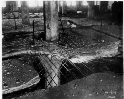
ILLUSTRATES HOW THE CONCRETE IS BEING PICKED TO PIECES IN ORDER TO DESTROY THE SLABS
