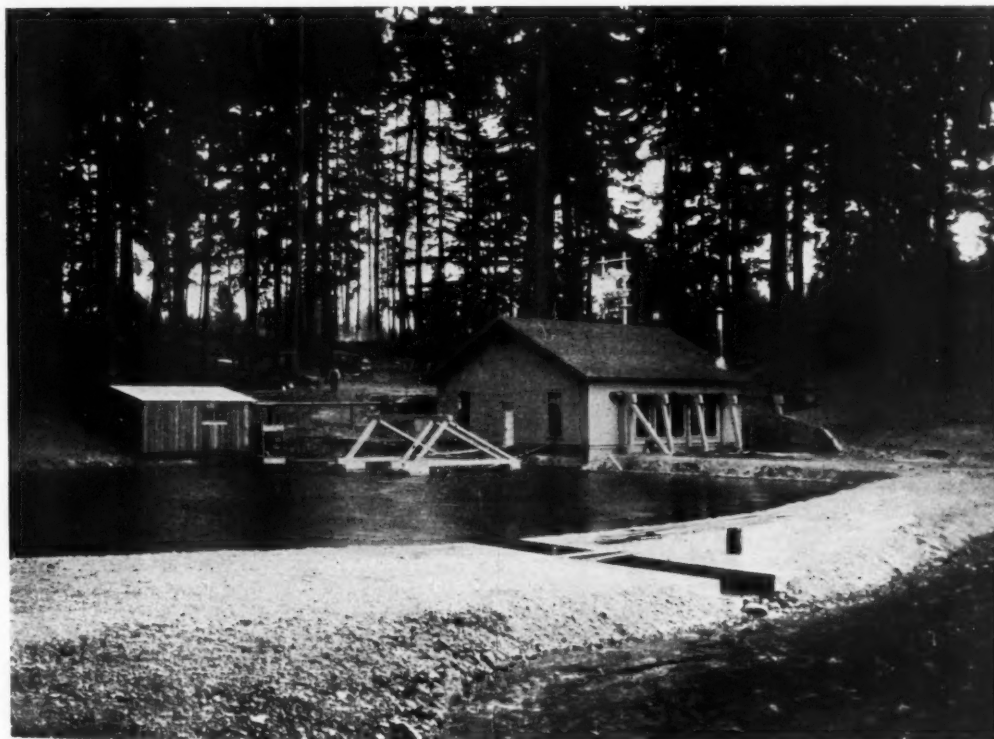
ONE OF THE PUMPING STATIONS
