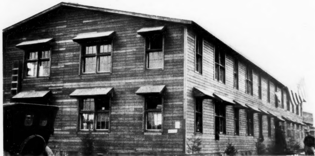
ONE OF THE TWO HUNDRED AND FIFTY BARRACK BUILDINGS FOR ACCOMMODATION OF TWO HUNDRED MEN EACH
