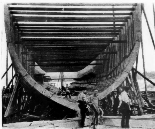
DOUGLAS FIR AS USED IN SHIP BUILDING IN BRITISH COLUMBIA
