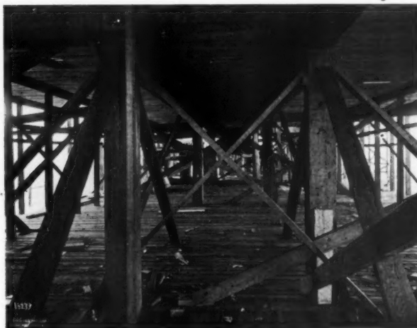
DOUGLAS FIR AS USED IN THE CONSTRUCTION OF A MILL BUILDING
