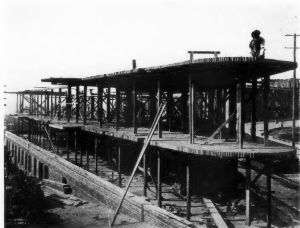
DOUGLAS FIR IN APARTMENT HOUSE CONSTRUCTION
