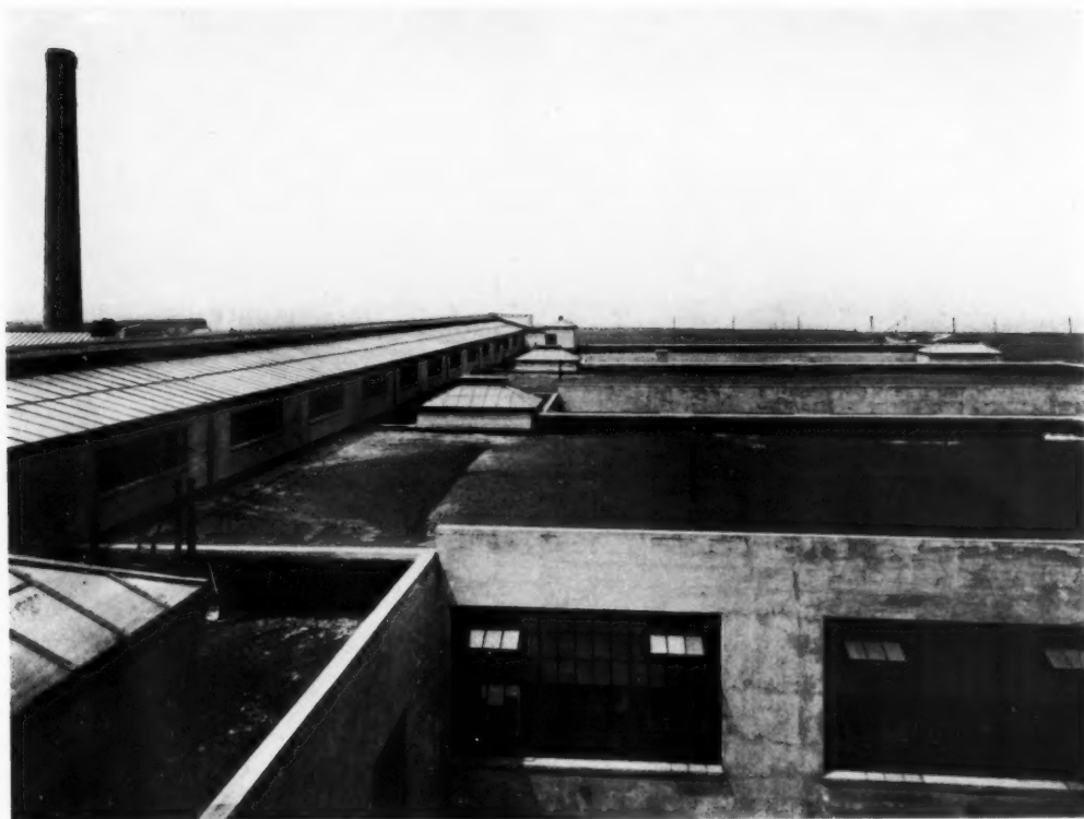
VIEW OF ROOF
