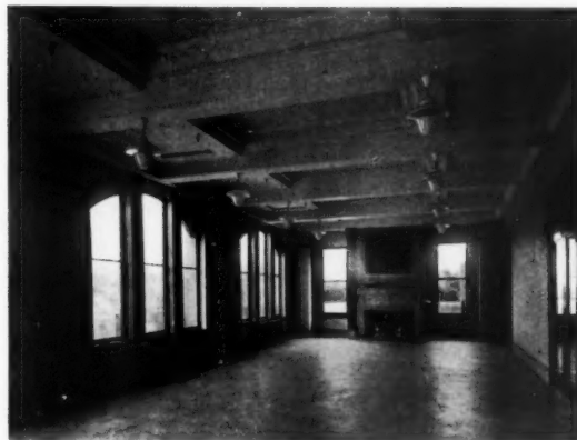
INTERIOR, ADMINISTRATION BUILDING
