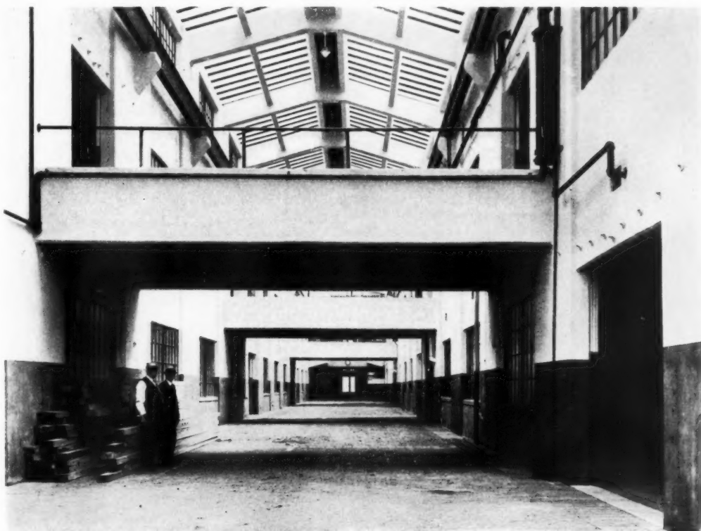
CRANEWAY—FIRST FLOOR (HEAD ROOM 12 FEET)
