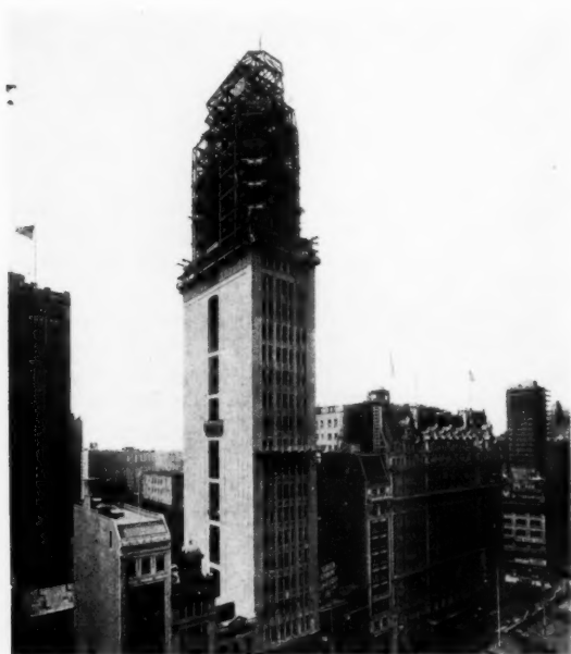
PROGRESS PHOTOGRAPH MAY 14, 1917. ALL STEEL IN PLACE AND WALLS COMPLETED TO THE 18TH FLOOR.
