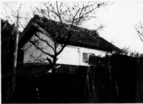
A FIREPROOF STORAGE VAULT
