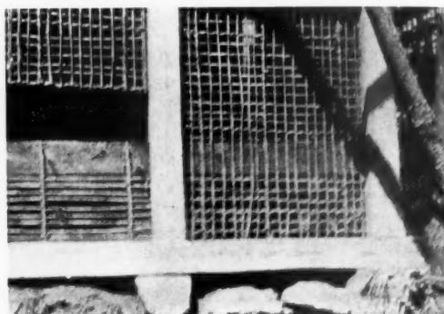
SHOWING THE STYLE OF LATH TO RECEIVE PLASTER. THIS IS MERELY STRIPS OF SPLIT BAMBOO
