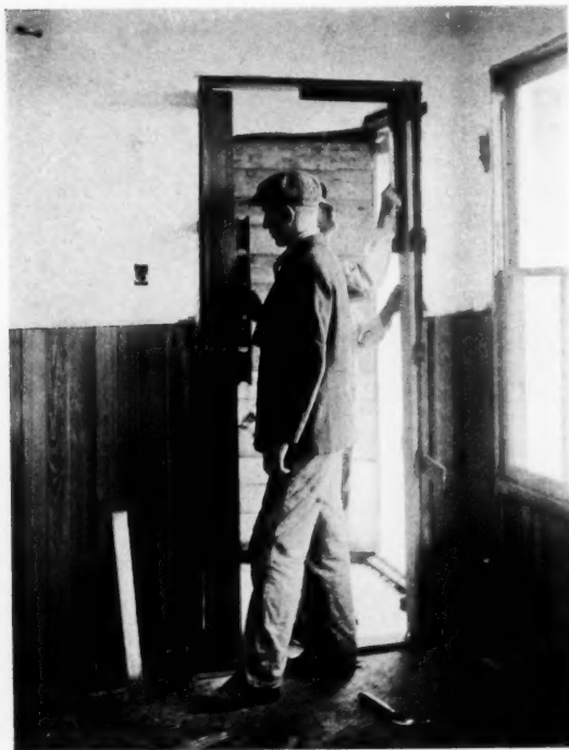
DOOR FRAMING—STATE TRADE SCHOOL, SOUTH MANCHESTER, CONN
