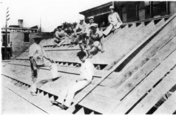
CARPENTERS—LATHROP SCHOOL OF MECHANICAL TRADES, KANSAS CITY, MO.
