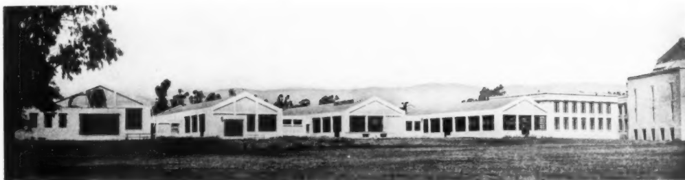
REAR VIEW OF SHOPS
