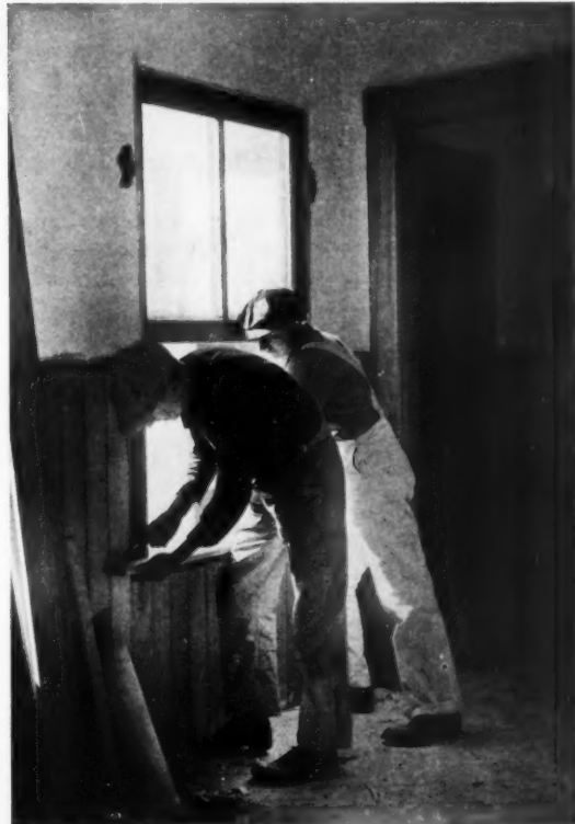
FITTING WINDOW FRAMES—STATE TRADE SCHOOL, SOUTH MANCHESTER, CONN.
