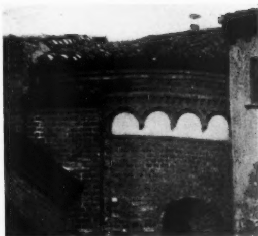
South transept end of S. Sepolcro at Milan, dating 1100. Showing a cornice with round arched corbel table of developed style.
