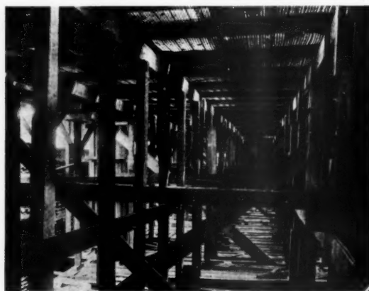
FIG. 5—VIEW OF FALSE-WORK, SHOWING METAL LATH ABOVE FOR FLAT CEILING
