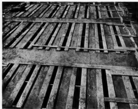
FIG. 4—CONCRETE POURED. FORMS NOT YET REMOVED
