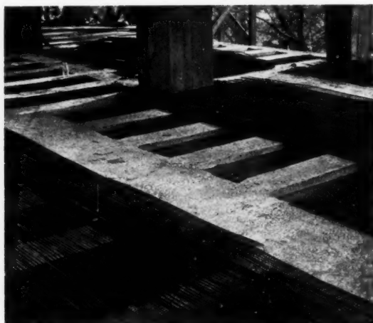
FIG. 6—FORMS REMOVED. EXPANDED METAL REINFORCEMENT FOR FLOOR FILL PARTIALLY LAID
