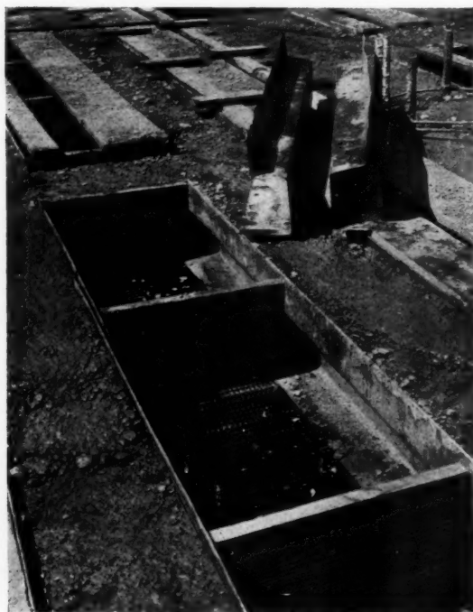
FIG. 7—FORMS AND SPACERS IN PLACE. NOTE STEEL FORMS ON TOP OF FLOOR
