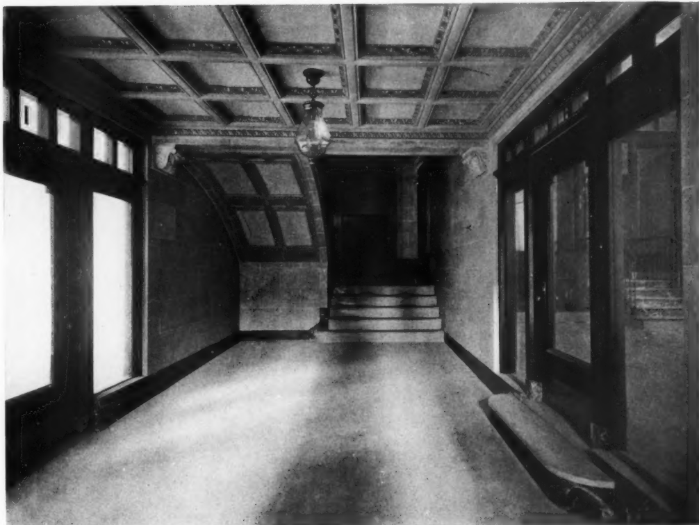
ENTRANCE HALL, TREMONT STREET
