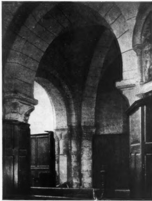
LOMBARD TYPE OF RIB VAULTING WITH HEAVY DIAGONAL RECTANGULAR RIBS
