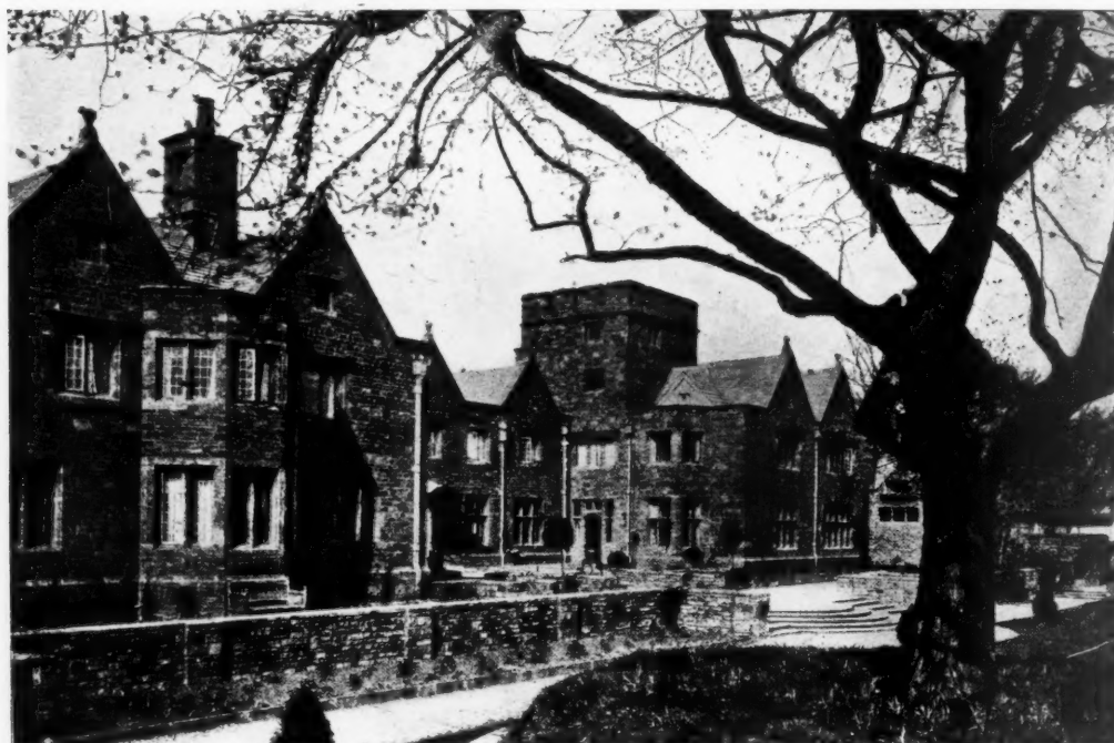
LITTLECOURT, FARTHINGSTONE, NORTHAMPTONSHIRE: TERRACE FRONT
