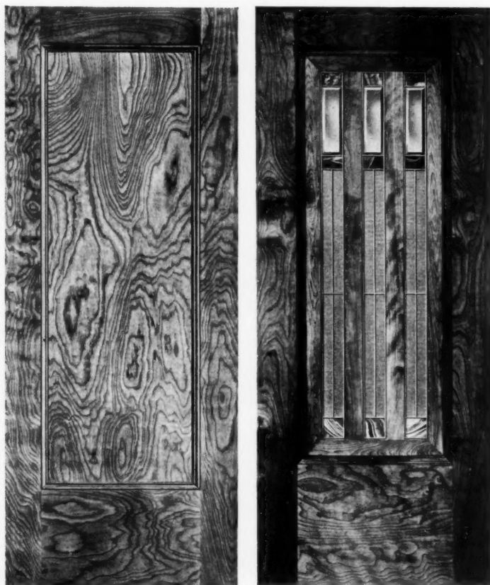
AT LEFT: FIGURED BIRCH, ROTARY CUT, SHOWING CONTOUR OR LANDSCAPE EFFECT. AT RIGHT: BIRCH VENEER, ROTARY CUT
