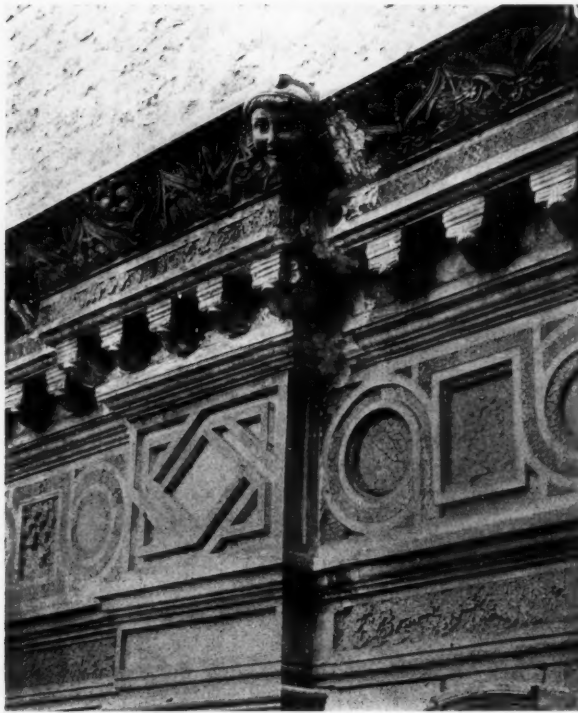
FIG. 12—DETAIL OF THE CORNICE OF THE LATERAN CLOISTER.
