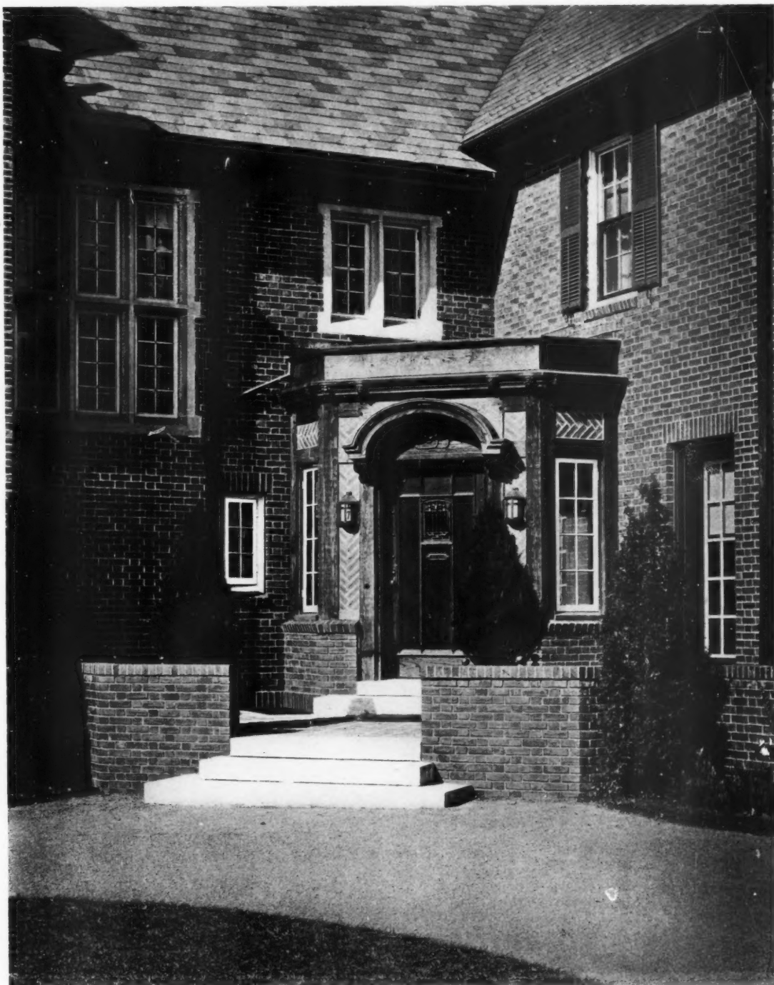
DETAIL OF ENTRANCE
