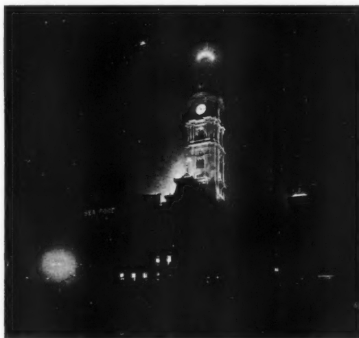
NEAR VIEW, TOWER OF CITY HALL, PHILADELPHIA
