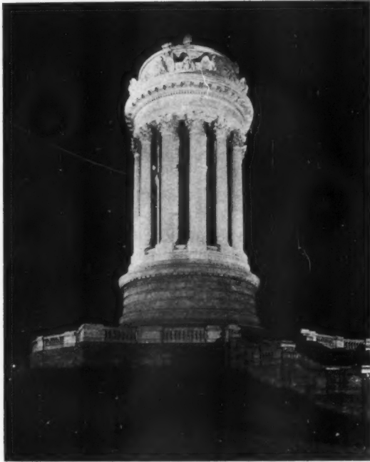
FLOOD LIGHTING OF SOLDIERS AND SAILORS MONUMENT, RIVERSIDE DRIVE, NEW YORK
