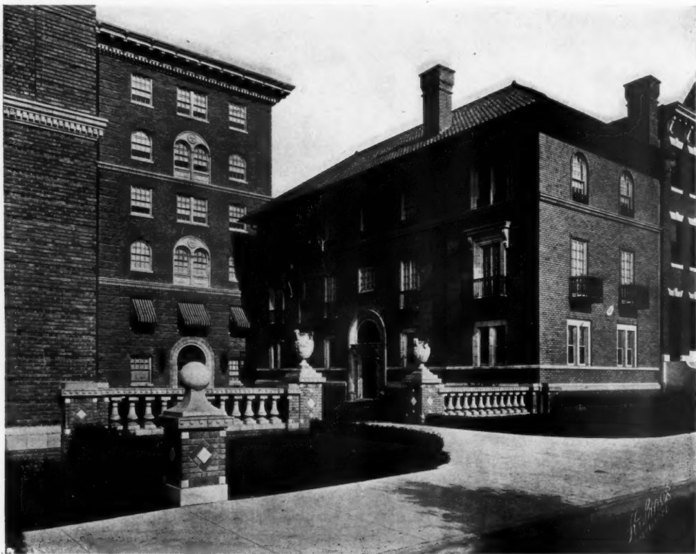
ADDITION TO HOMEWOOD APARTMENTS
