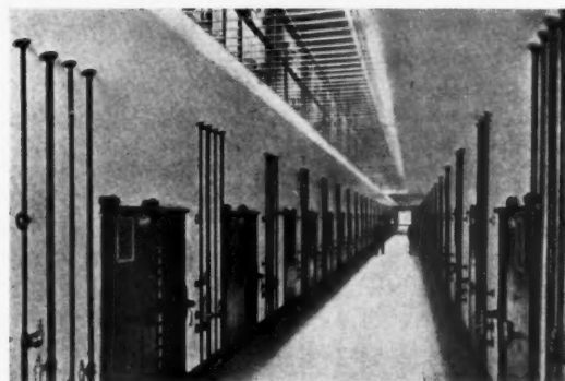
INTERIOR OF NEW CELL BLOCK EASTERN PENNSYLVANIA PENITENTIARY
