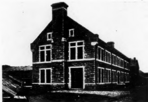
INDUSTRIAL BUILDING EASTERN PENNSYLVANIA PENITENTIARY
