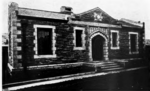
EMERGENCY HOSPITAL EASTERN PENNSYLVANIA PENITENTIARY
