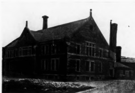
STORE HOUSE EASTERN PENNSYLVANIA PENITENTIARY
