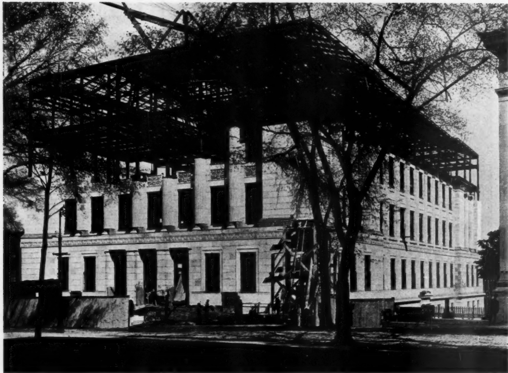
EAGLE STREET FAÇADE DURING CONSTRUCTION
