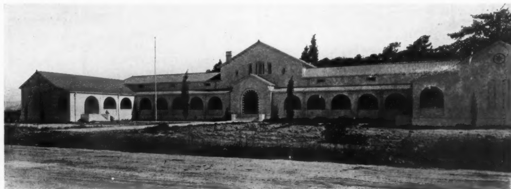
GARVEY AVENUE SCHOOL, ALHAMBRA, CAL.
