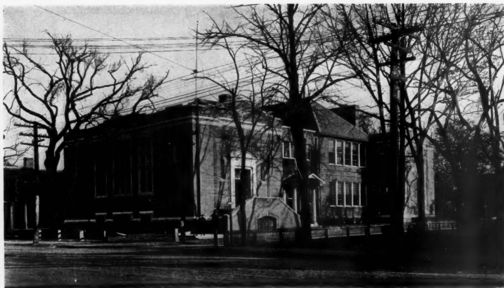
THOMAS HILL SCHOOL, WALTHAM, MASS. MESSRS. BRAINERD & LEEDS, ARCHITECTS
