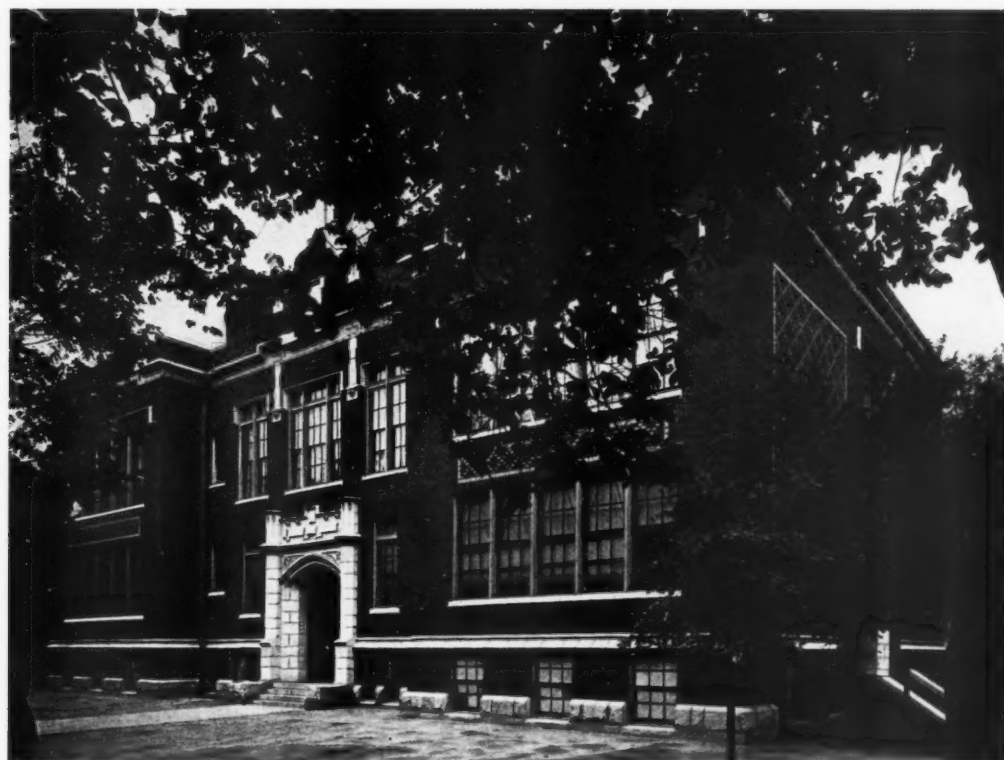
CREW STREET SCHOOL, ATLANTA, GA.
