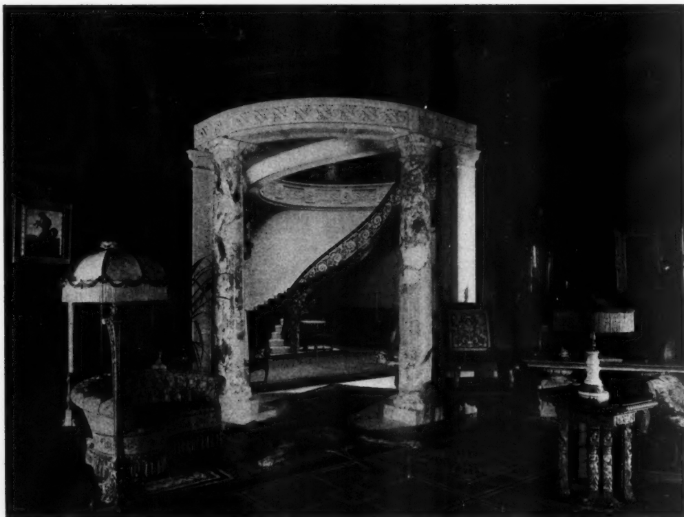
LIVING ROOM LOOKING TOWARD MAIN HALL
