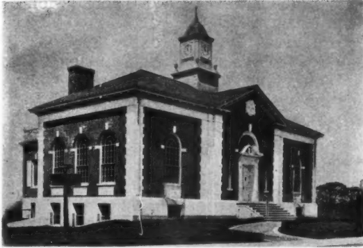
NEEDHAM PUBLIC LIBRARY, NEEDHAM, MASS. JAMES H. RITCHIE, ARCHITECT
