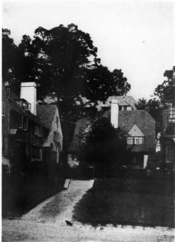
DETAIL, KENSINGTON TERRACE
