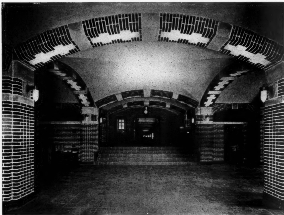
DETAIL OF MAIN LOBBY
