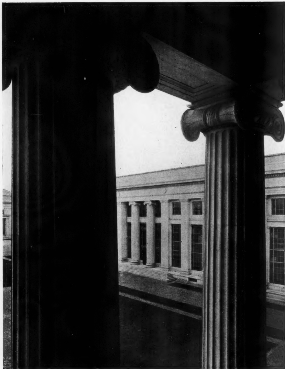
DETAIL OF COLUMNS, ENTRANCE PORTICO
