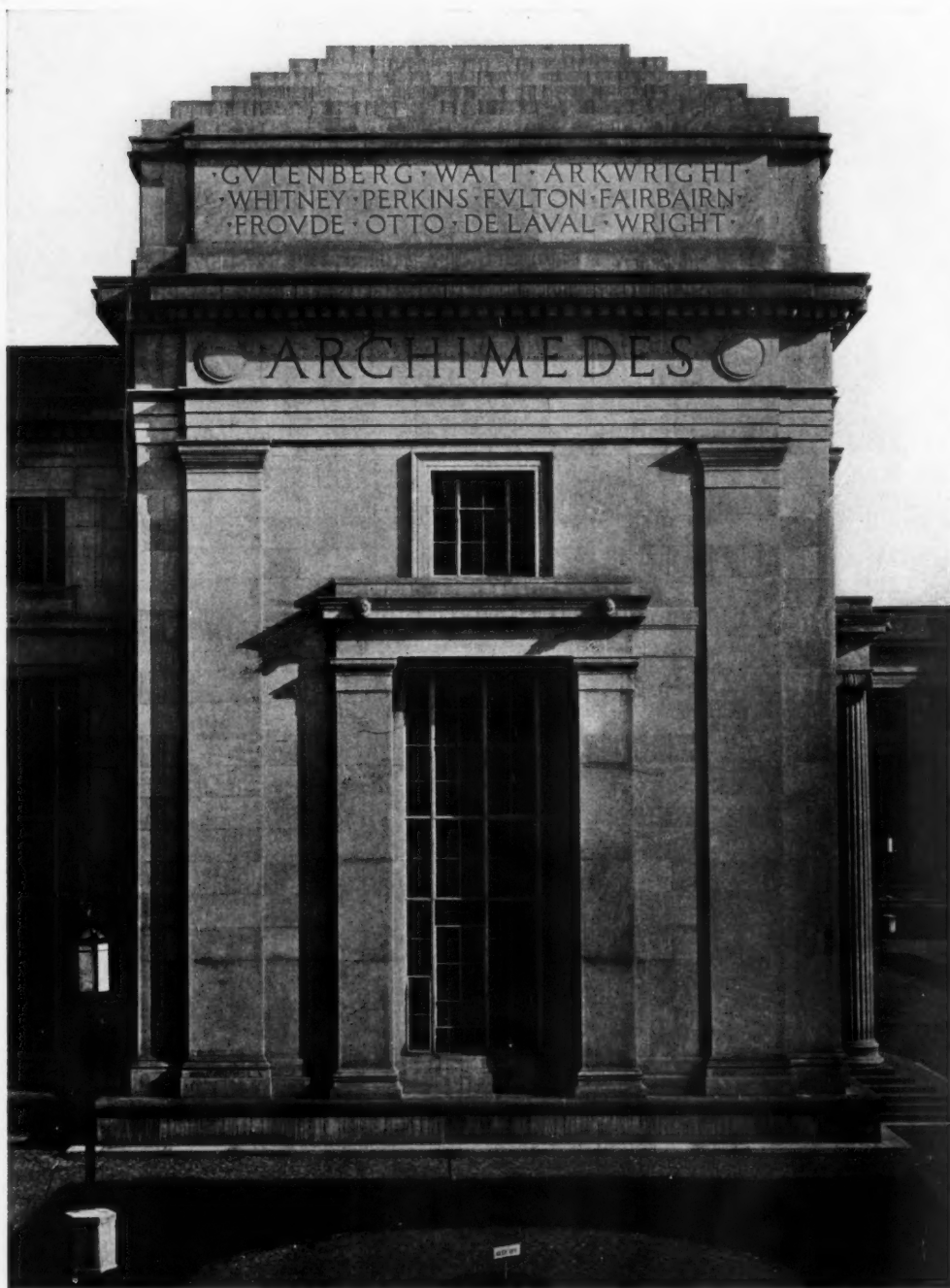
DETAIL OF PAVILION AT CORNER BETWEEN MAIN COURT AND MINOR COURT NEW BUILDINGS, MASSACHUSETTS INSTITUTE OF TECHNOLOGY, CAMBRIDGE, MASS.
