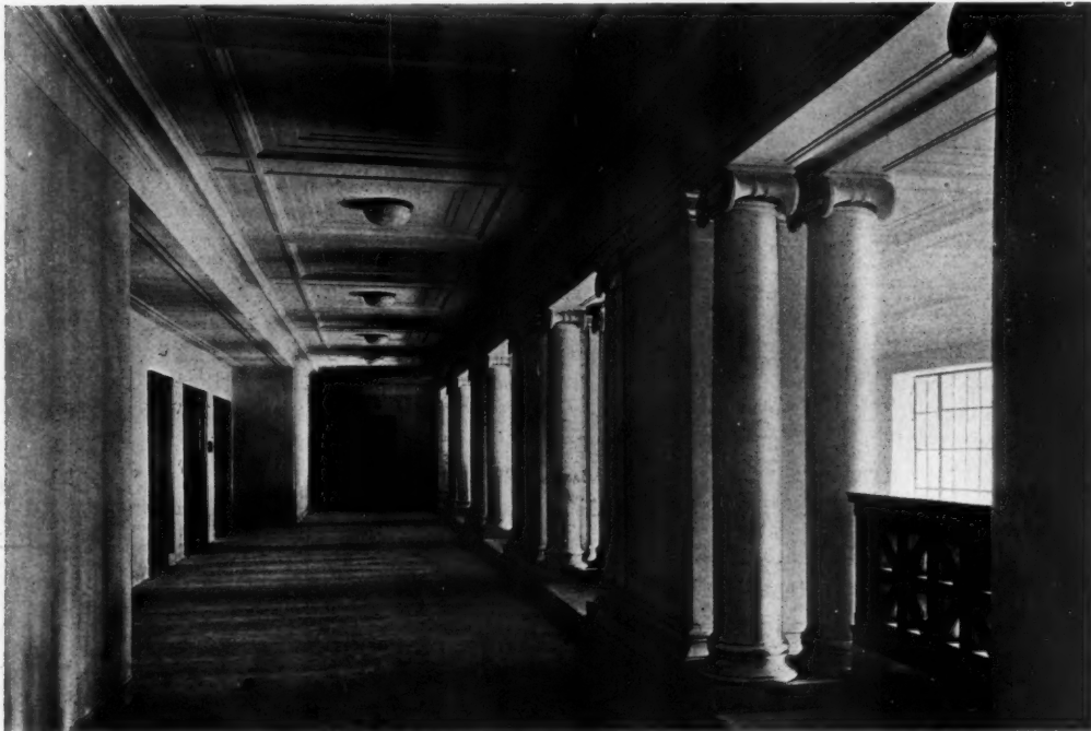
VIEW SHOWING CORRIDOR TREATMENT IN MAIN BUILDING
