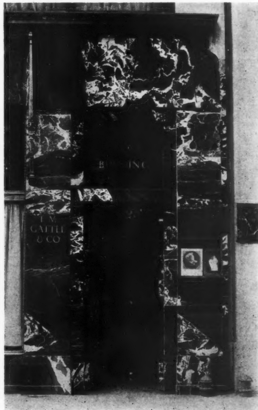
GRAND ANTIQUE MARBLE ENTRANCE, CLEWS BUILDING, NEW YORK MESSRS. STARRETT & VAN VLECK, ARCHITECTS
