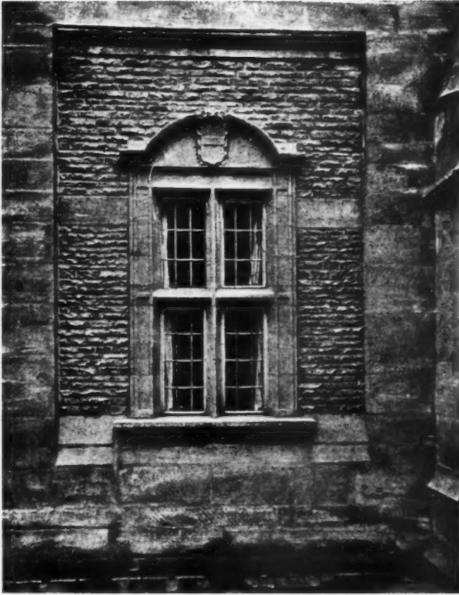
DETAIL OF A WINDOW IN PORTER'S LODGE, EMMANUEL COLLEGE, CAMBRIDGE, ENGLAND
