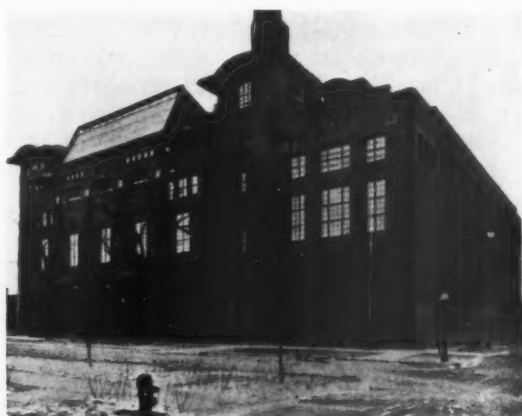
GENERAL VIEW FROM NORTH, Y. M. C. A. COLLEGE, CHICAGO
