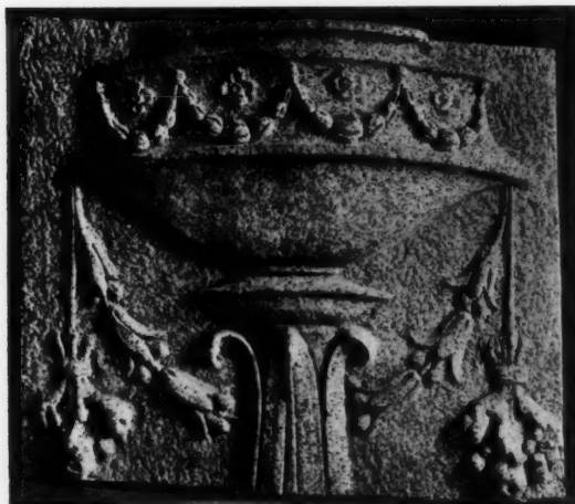
UNGLAZED "GRANITE" TERRA COTTA WITH ORNAMENT SMOOTH AND BACKGROUND LIGHTLY BUSH-HAMMERED
