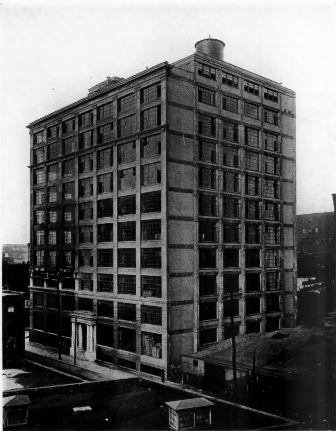
KENT BUILDING, BROOKLYN, N. Y. MESSRS. DAY & ZIMMERMAN, ARCHITECTS AND ENGINEERS
