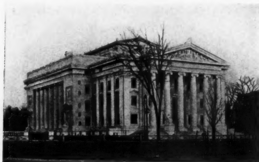
COUNTY COURT HOUSE, NEW HAVEN, CONN.
