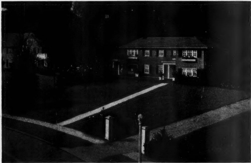
NO. 6. WOODEN HOUSE MODEL WITH REGULATION GLASS IN WINDOWS. NOTE PLANTINGS (See Lot No. 4, Figure No. 1)
