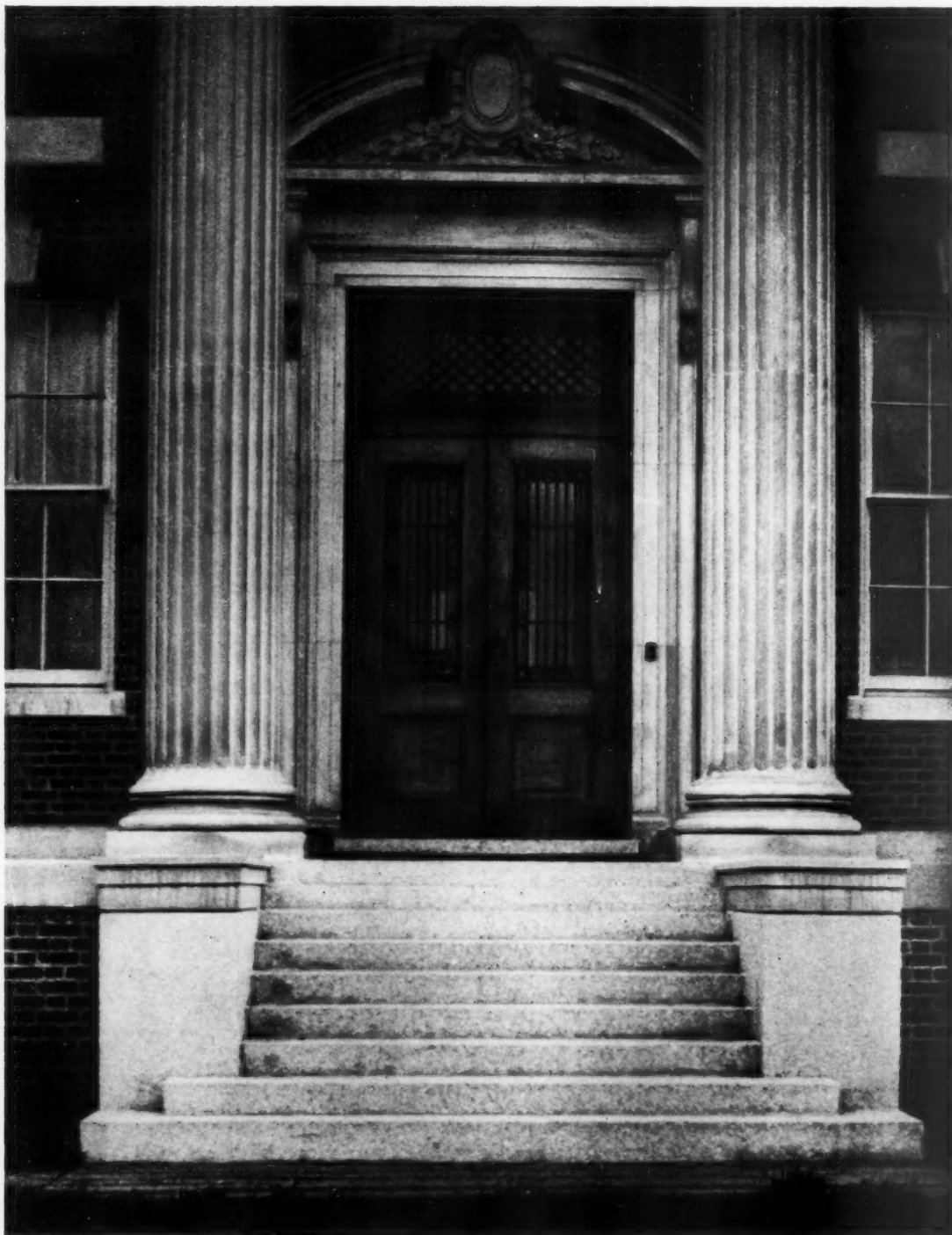
DETAIL OF ENTRANCE
