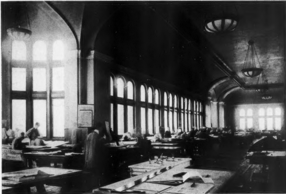
A VIEW IN THE NEW DRAUGHTING ROOM THIS ROOM IS NEARLY 200 FEET LONG AND CONTAINS 190 TABLES, IDEALLY LIGHTED
