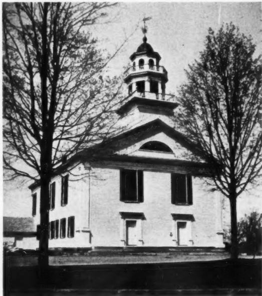
CONGREGATIONAL CHURCH, HOLLIS, N. H.
