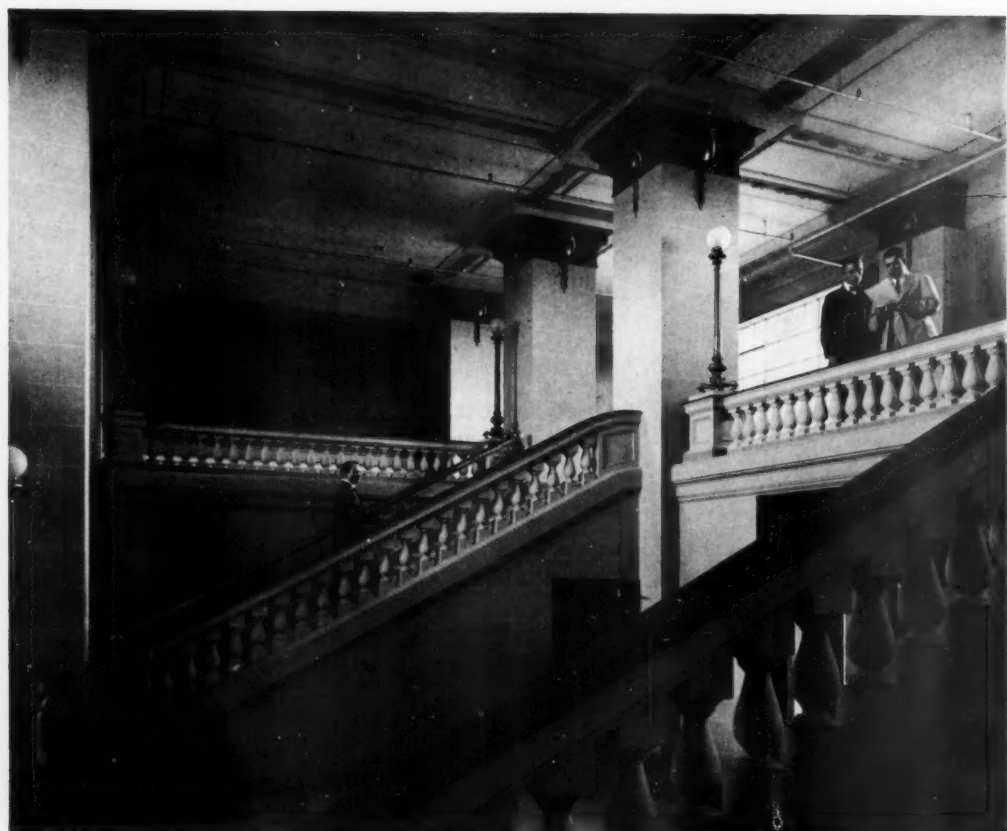
DETAIL OF STAIRWAY BROWN & BIGELOW BUILDING, ST. PAUL, MINN. MESSRS. KEES & COLBURN, ARCHITECTS
