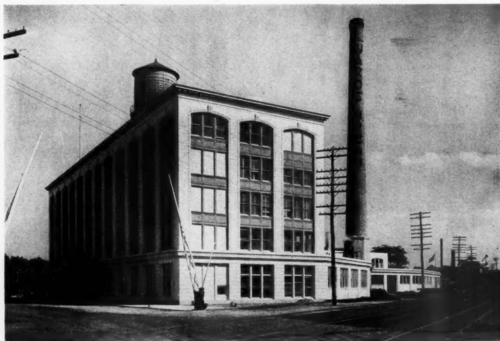
BAKERY BUILDING—WARD BREAD CO., AMPERE, N. J.
