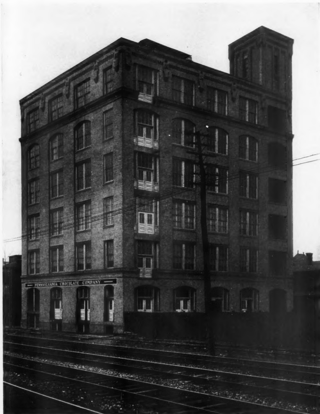
PENNSYLVANIA CHOCOLATE CO.'S BUILDING, PITTSBURGH, PA.
