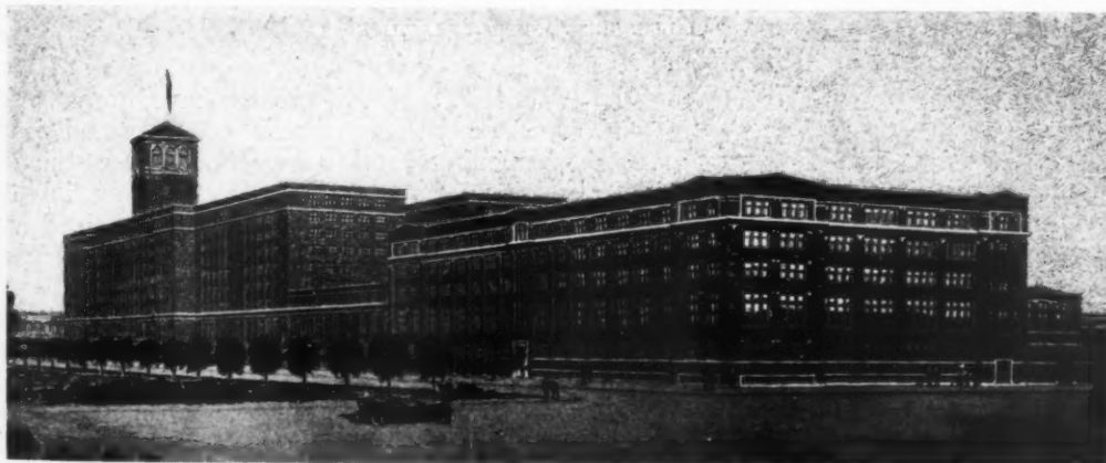
GROCERY DEPARTMENT BUILDING: SEARS, ROEBUCK & CO., CHICAGO, ILL.
