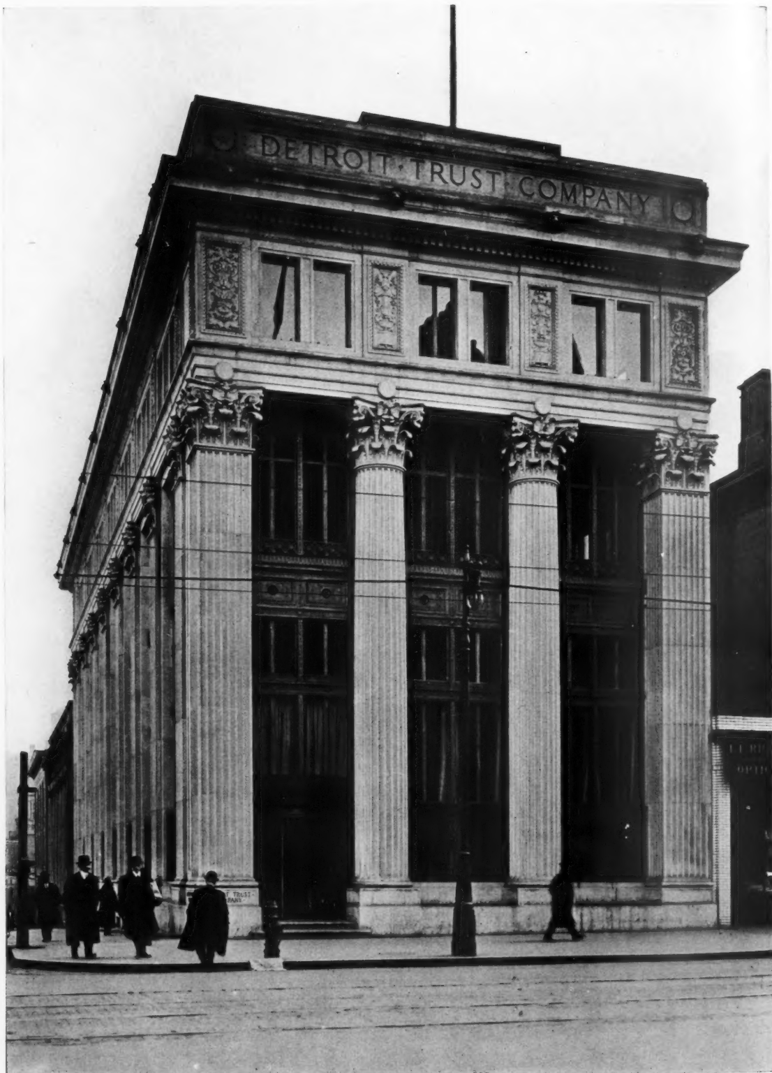
BUILDING FOR DETROIT TRUST CO., DETROIT, MICH.
