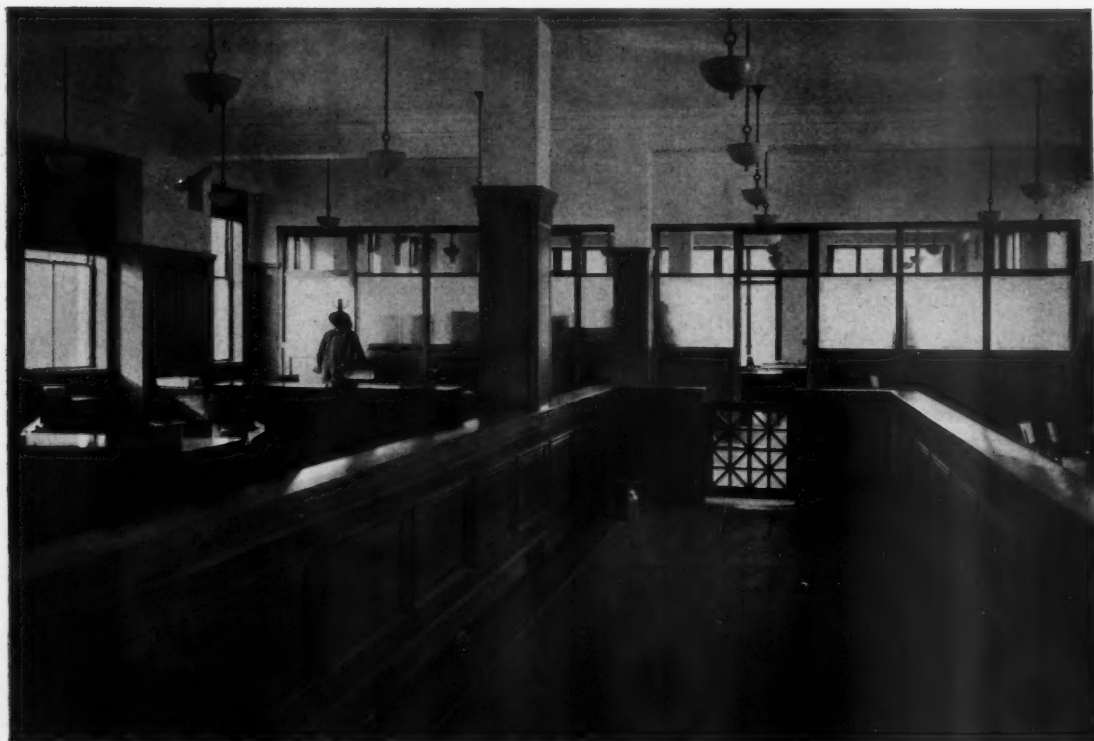
OFFICES ON SECOND FLOOR
