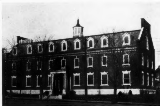
POLICE HEADQUARTERS BUILDING, MOUNT VERNON, N. Y.
