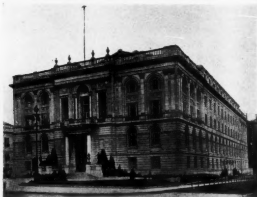
MUNICIPAL BUILDING, HARTFORD, CONN.
