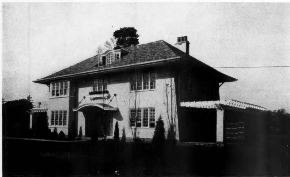
HOUSE AT LATHAM PARK, PA.
