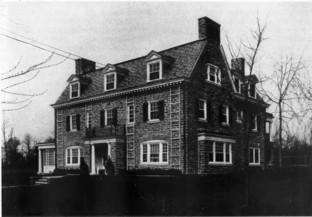
HOUSE AT GREEN LANE MANOR, PHILADELPHIA, PA.
