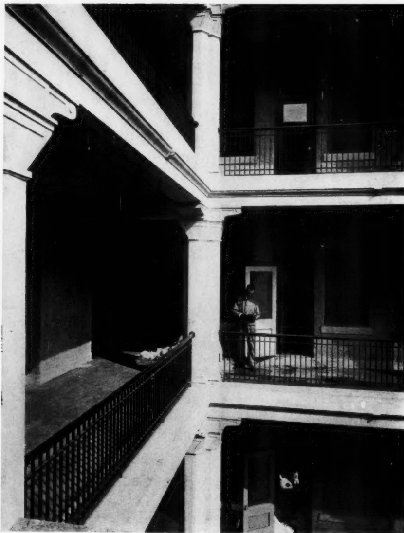
GALLERIES, ISOLATION WARD
