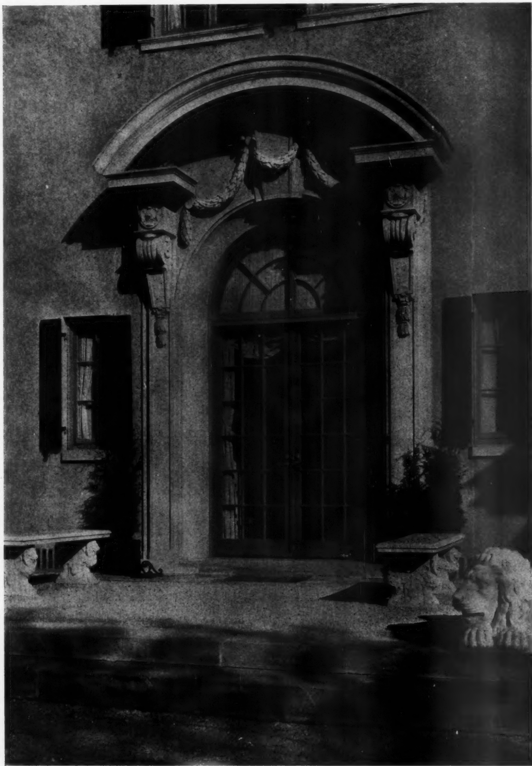
DETAIL OF MAIN ENTRANCE
