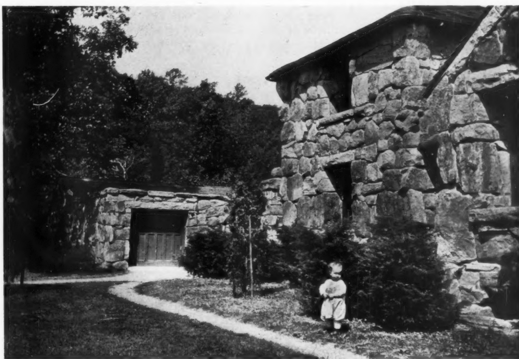
GATE LODGE FOR FRANCIS L. STETSON, ESQ., STERLINGTON, N. Y.
