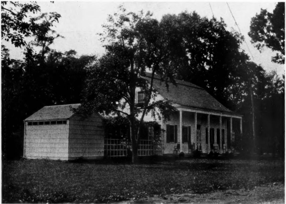
SUPERINTENDENT'S COTTAGE, ESTATE OF GLENN STEWART, ESQ., LOCUST VALLEY, L. I.
