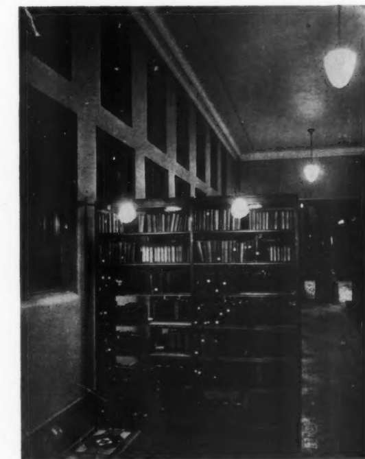
FIG. 5. SHOWING ARRANGEMENT FOR LIGHTING BOOK STACKS
