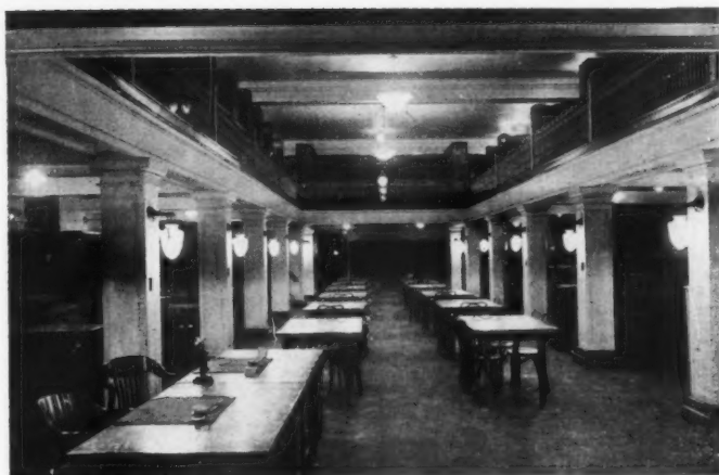
FIG. 4. A UNIQUE AND PLEASING ARRANGEMENT OF WALL BRACKETS THAT DOES AWAY WITH TABLE LAMPS
