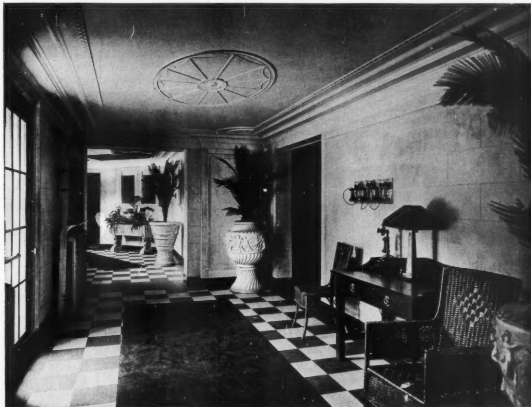
ENTRANCE HALL, HARDY APARTMENTS
