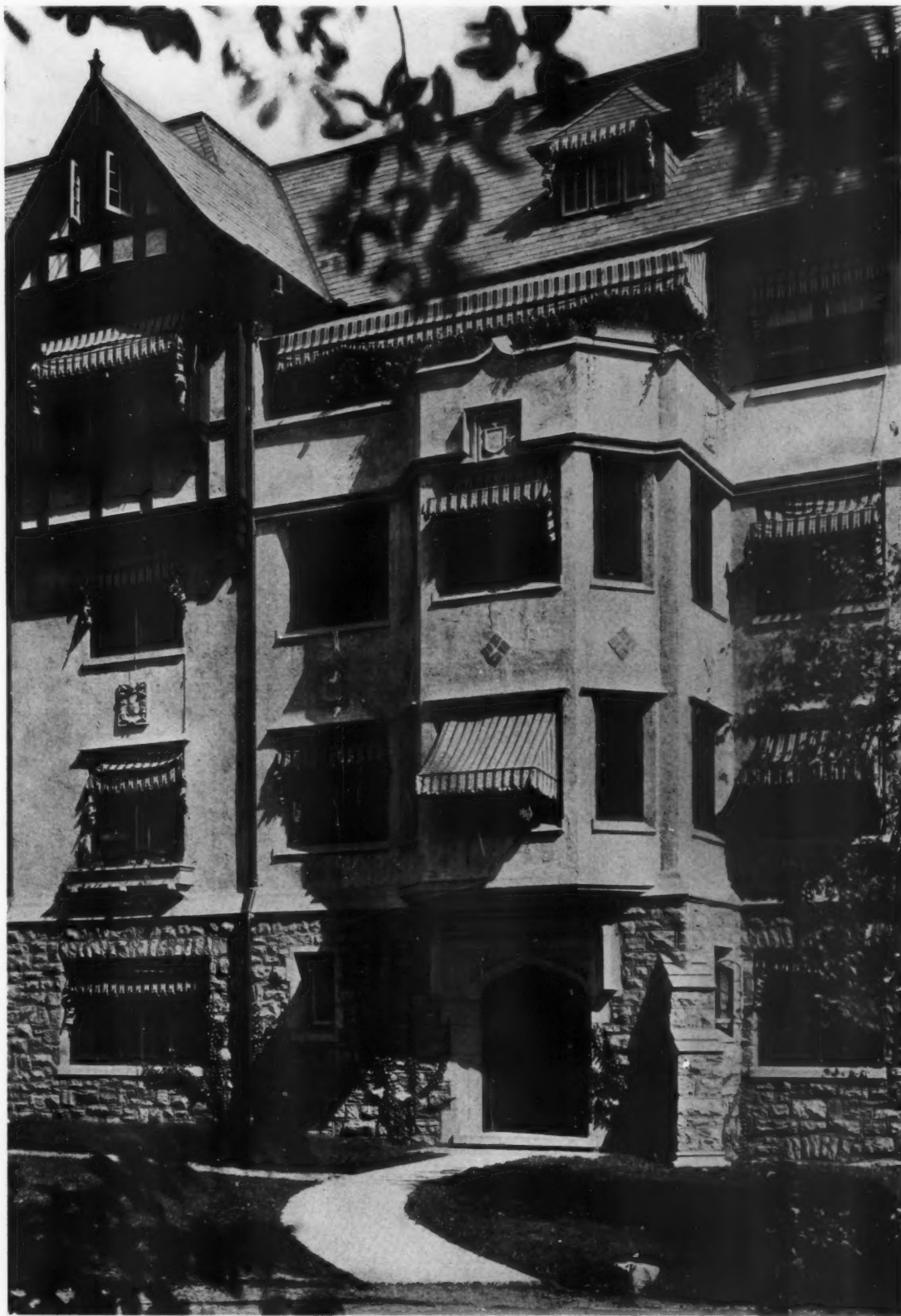
ENTRANCE DETAIL, HOUSE NO. 3
