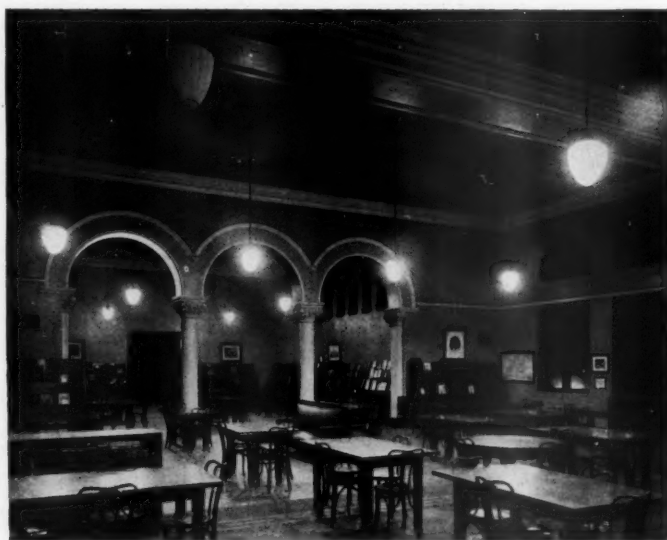
FIG. 3. PENDANT FIXTURES ILLUMINATING THE REFERENCE ROOM
