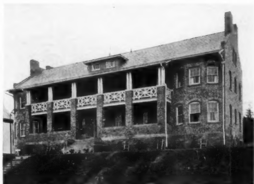
U. S. Army Officers' Quarters, Fort Worden, Wash. Floors soundproofed with Hydrex-SANIFLOR.
