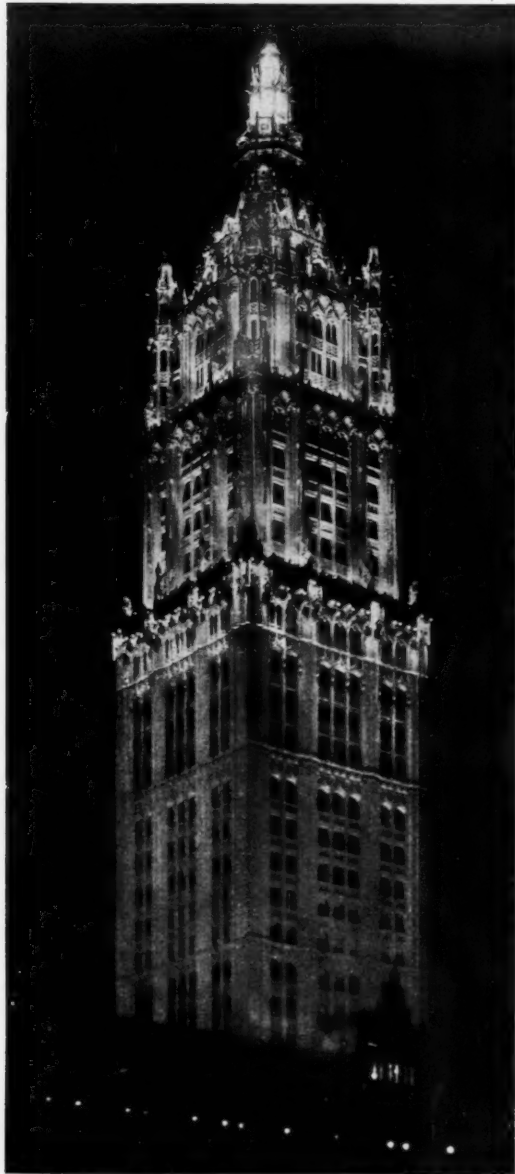
WOOLWORTH TOWER, NIGHT VIEW. TWENTY 1,000 C.P. LAMPS IN LANTERN SO DIFFUSED THAT NO INDIVIDUAL POINT OF LIGHT IS VISIBLE
