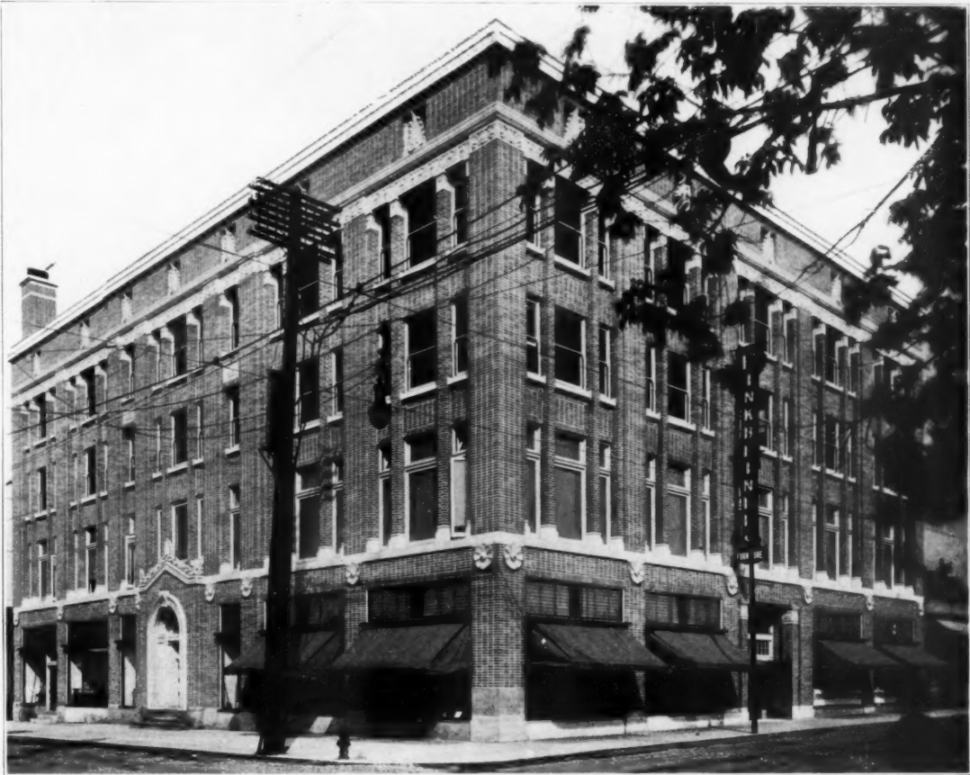
YONDOTA MASONIC TEMPLE, TOLEDO, OHIO. Mills, Rhines, Bellman & Nordhoff, Architects.
