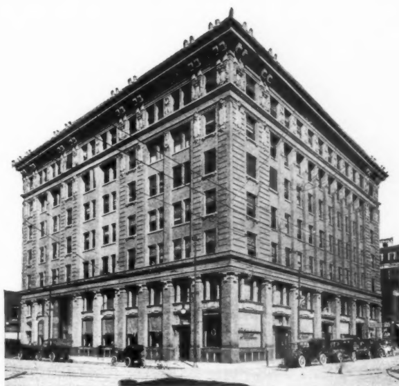
First National Bank, El Paso, Tex. Frost & Frost, El Paso, Architects Kewanee Smokeless installed by The Elliott Engineering Co.
