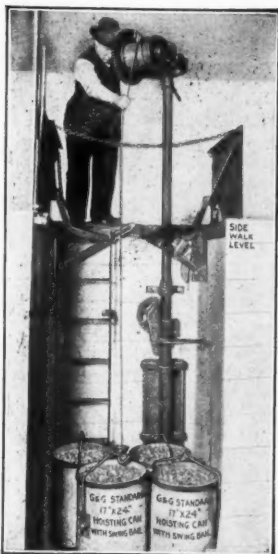
Illustration also shows the G & G Sidewalk Door Opening and Closing Device which automatically opens and closes doors as hoisting head is raised or telescoped.
