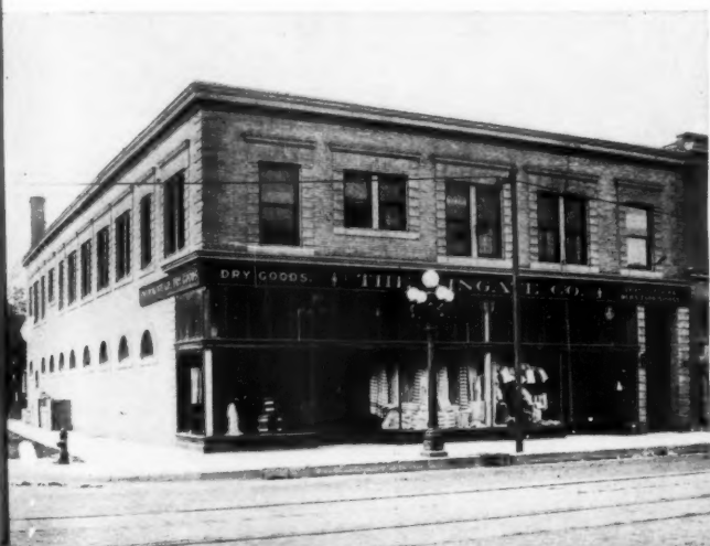
The Wingate Co., Minneapolis No. 106 Kewanee Smokeless Boiler Installed
