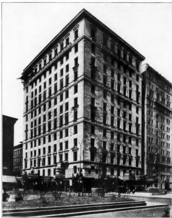
400 Park Avenue. Warren & Wetmore, Archts., Fullerton, Weaver Realty Co., Owners. 2 Kewanee Smokeless Boilers Installed by W.G. Cornell Co.
