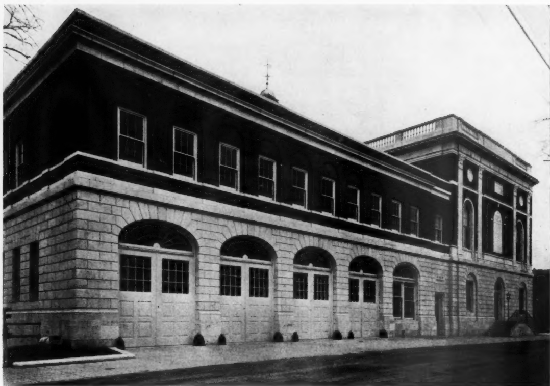
FIRE DEPARTMENT SECTION
