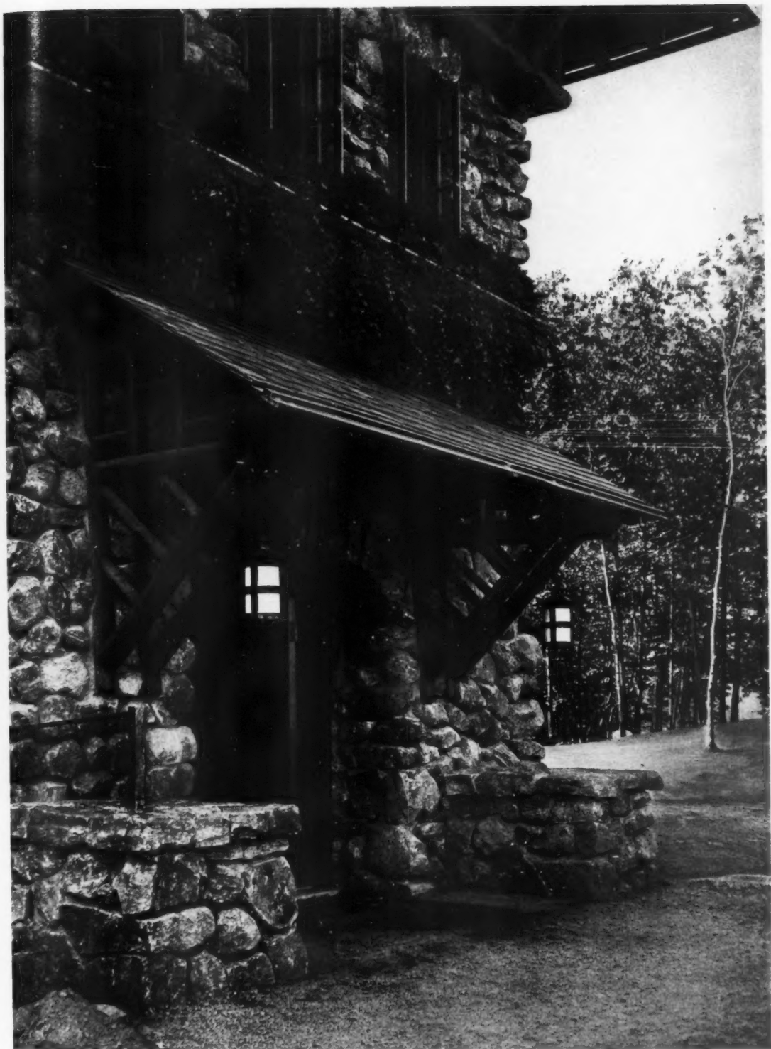
HEADQUARTERS BUILDING—PALISADES INTERSTATE PARK, BEAR MOUNTAIN, N. Y.
