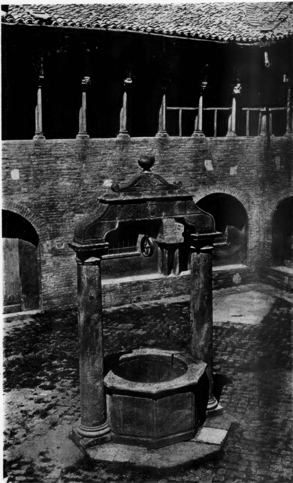
WELL CURB, SANTA STEFANO, BOLOGNA
