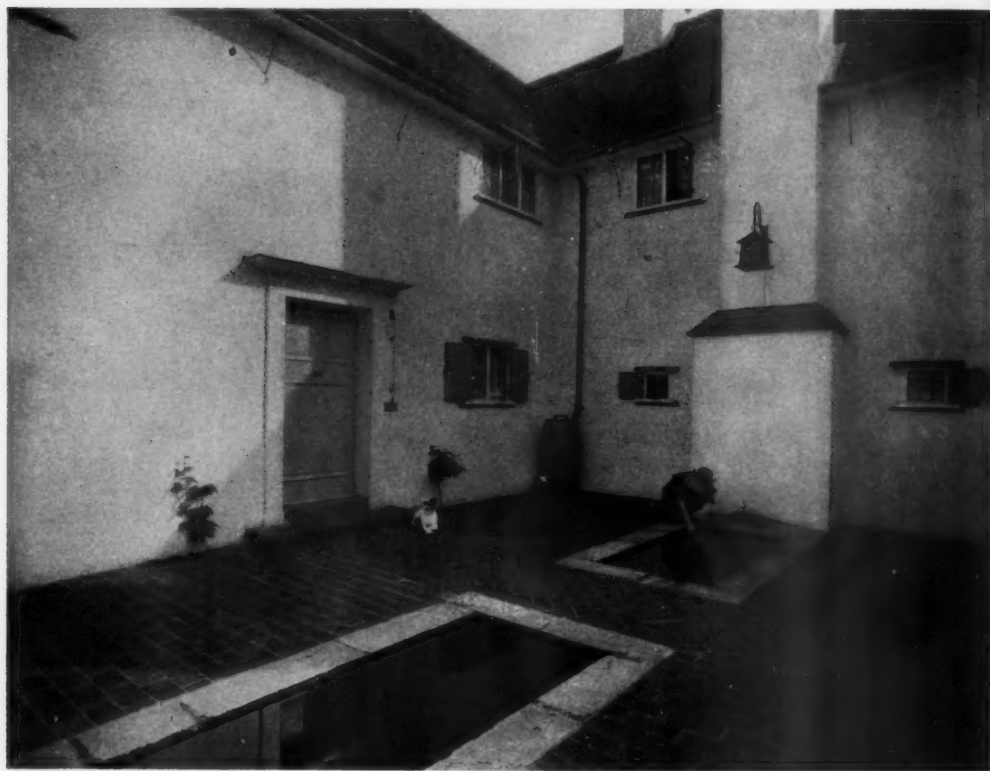
A COURTYARD IN A COUNTRY HOUSE
