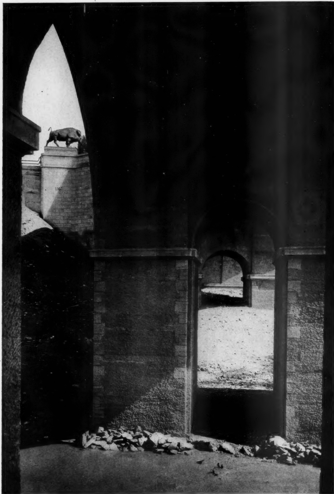
THE Q STREET BRIDGE, WASHINGTON, D. C. MESSRS. GLENN BROWN AND BEDFORD BROWN IV, ARCHITECTS
