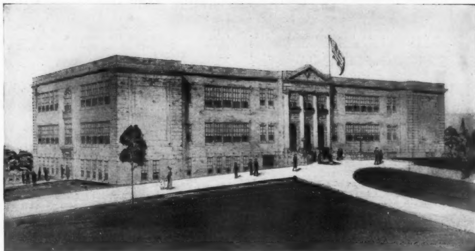
Ingram School, Pittsburgh, Pennsylvania Press C. Dowler, Pittsburgh, Architect. F. E. Geisler & Co., Heating Contractors. Kewanee Smokeless Boilers Installed
