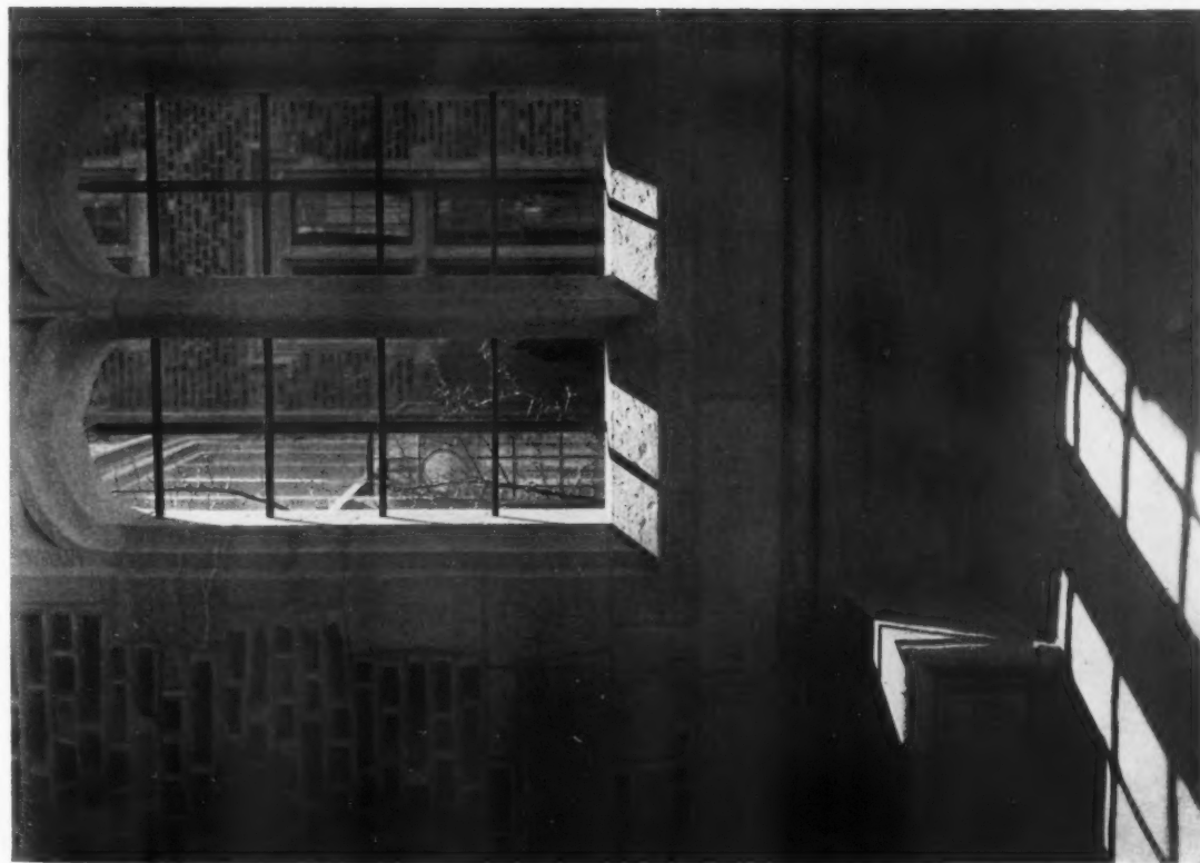
WINDOW IN TOWER ENTRANCE
