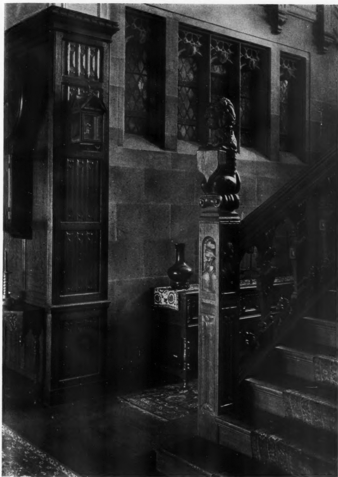
DETAIL OF MAIN STAIRCASE
